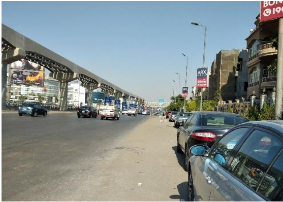
Figure 2-10 Photo taken showing monorail
