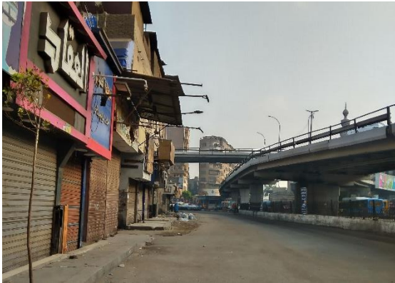
Figure 2-19 Photo showing street towards Mosque of Al-Qadi Yahya
