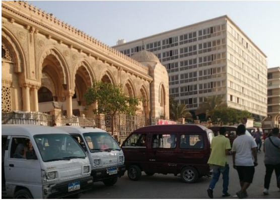
Figure 2-6 Photo taken Al-Hosary Mosque.
