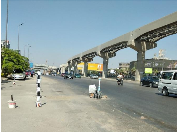
Figure 3-36 Image showing crossing situation along South 90th road
