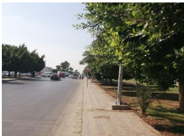
Figure 3-39 Image showing protection from weather situation
